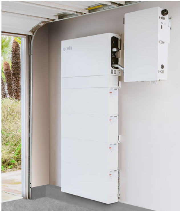
San Diego, CA homeowner installation
