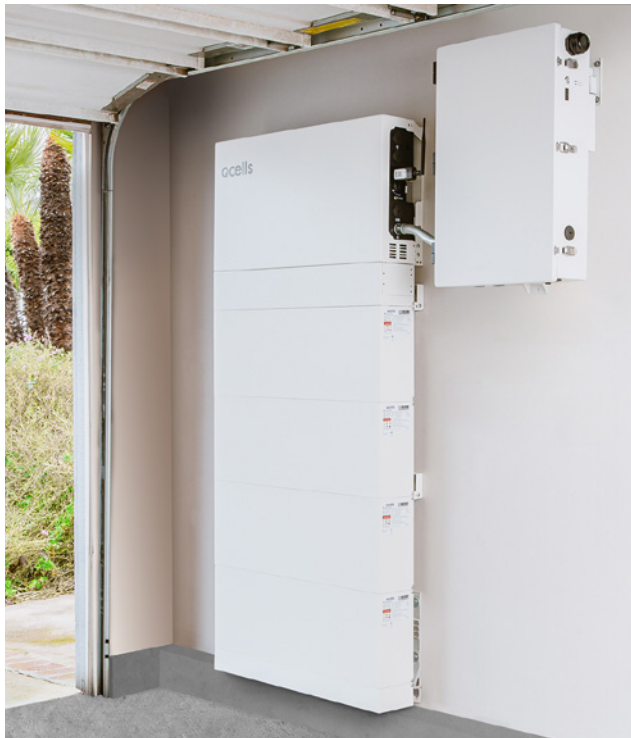
San Diego, CA homeowner installation
